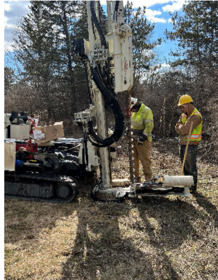
Geotechnical drilling occurring at the Yahara Hills Golf Course.
